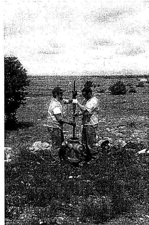
Operations Staff rebuilding fire hydrant
