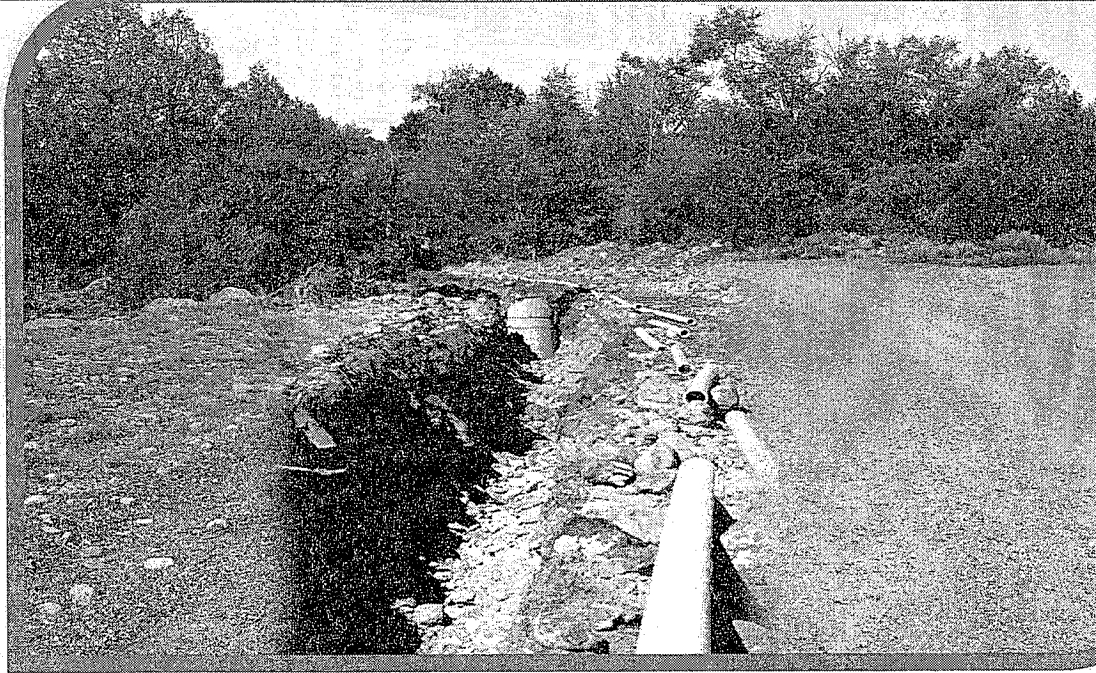
Antelope Way under construction - May 1981 Then and Now
