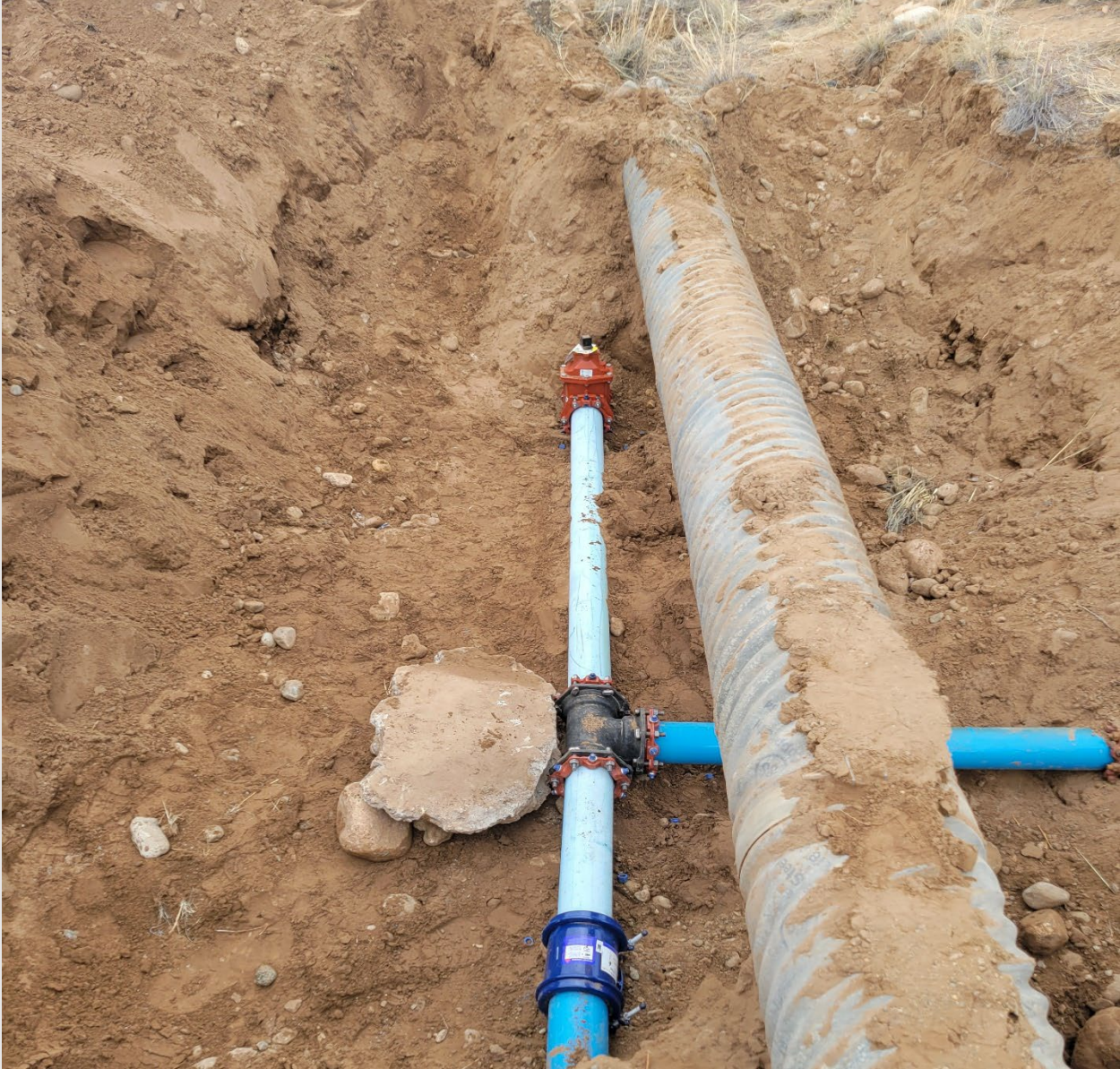
Main Repair on Peaceful way in November
