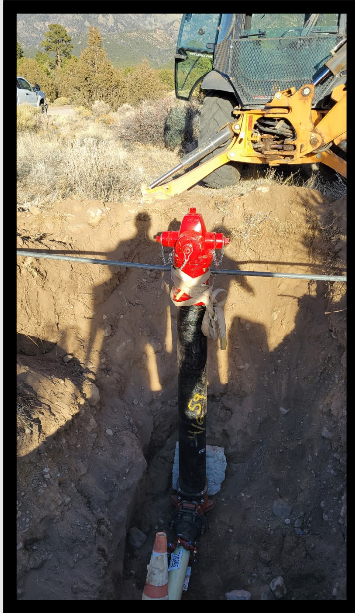
Fire Hydrant Replacement on Antelope
