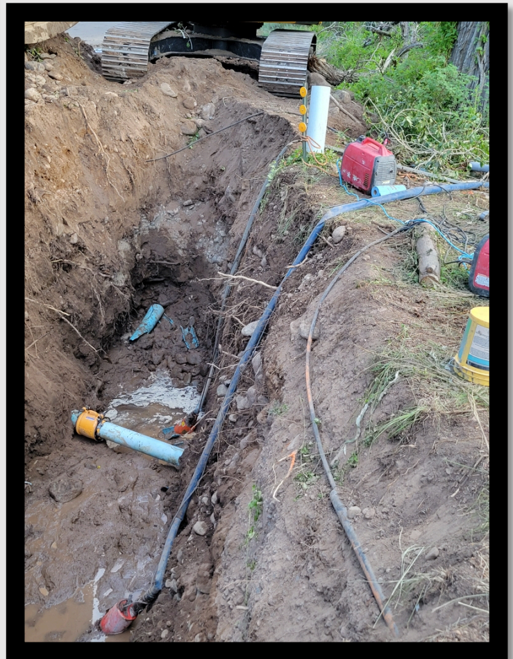
Picture of Wagon Wheel Forced Main Repair Near Spanish Creek 8/18/22
