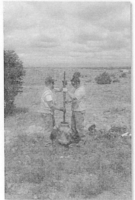
Operations Staff rebuilding fire hydrant
